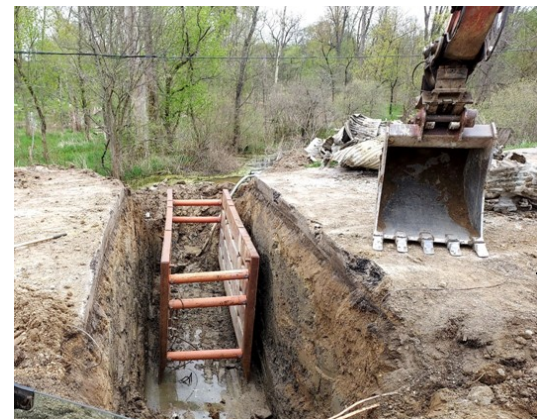
CR 64 culvert replacement
